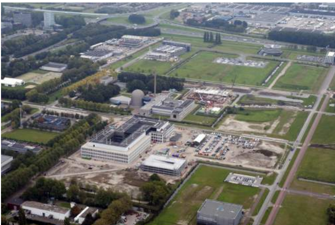
Figure 1: 2MW light water reactor for positrons, neutron scattering, activation analysis and isotope production research. A cold source for the experimental hall will be installed in 2018, feeding SANS, SESANS, TOF-reflectometer.
